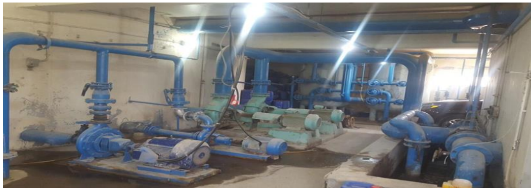
Water Conservation (Al-Furat Al-Awsat Technical University,IRAQ)
