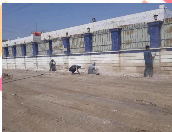
17. Implementation and clearing works on the institute's external fence.
