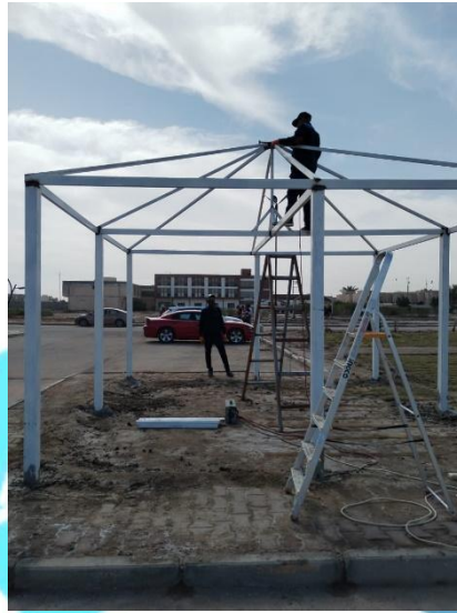
Implementation and clearing works on the institute's external fence..17
