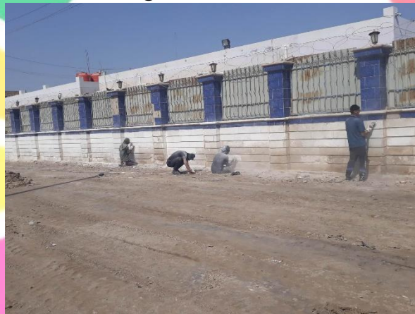
The final stages of construction work for the health laboratory annex..18
