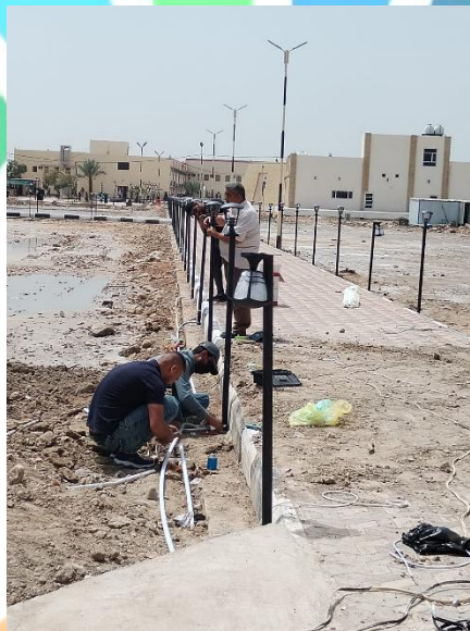
Implementation works for the external fountain of the Technical Institute..15
