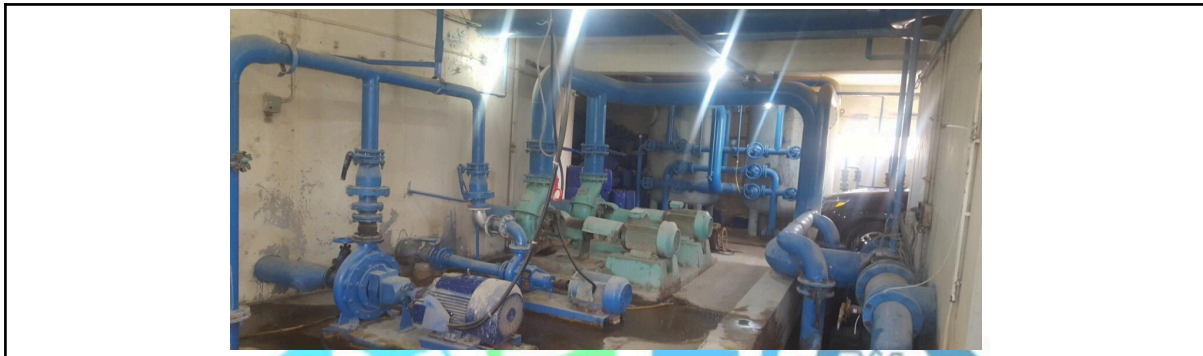
Water Conservation (Al-Furat Al-Awsat Technical University,IRAQ)
