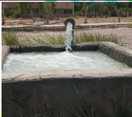
Water Conservation - In Ground Water Tank (Al-Furat Al-Awsat Technical University,IRAQ)
