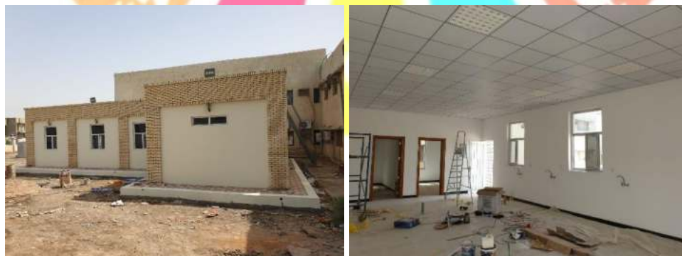
18. The final stages of construction work for the health laboratory annex.
