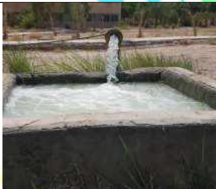
Water Conservation - In Ground Water Tank (Al-Furat Al-Awsat Technical University,IRAQ)
